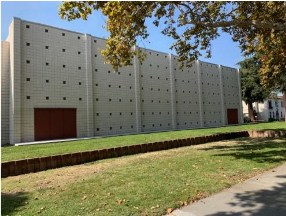
Figure 2. Partial east elevation showing exterior of large gymnasium
