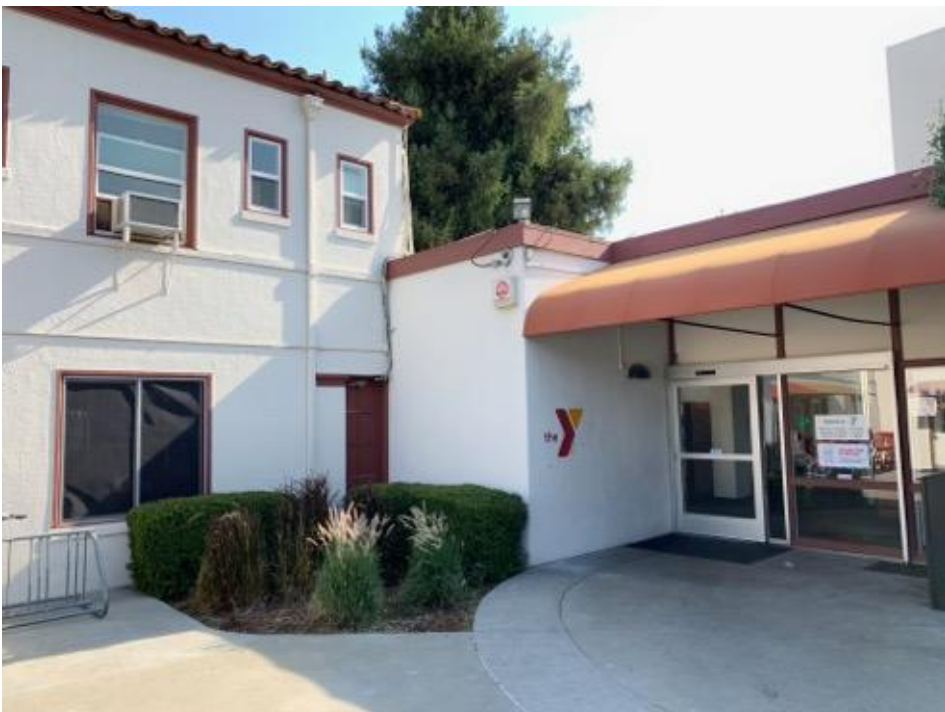
Figure 13. Partial west elevation of administration building (left) showing attachment to main YMCA facility (right)
