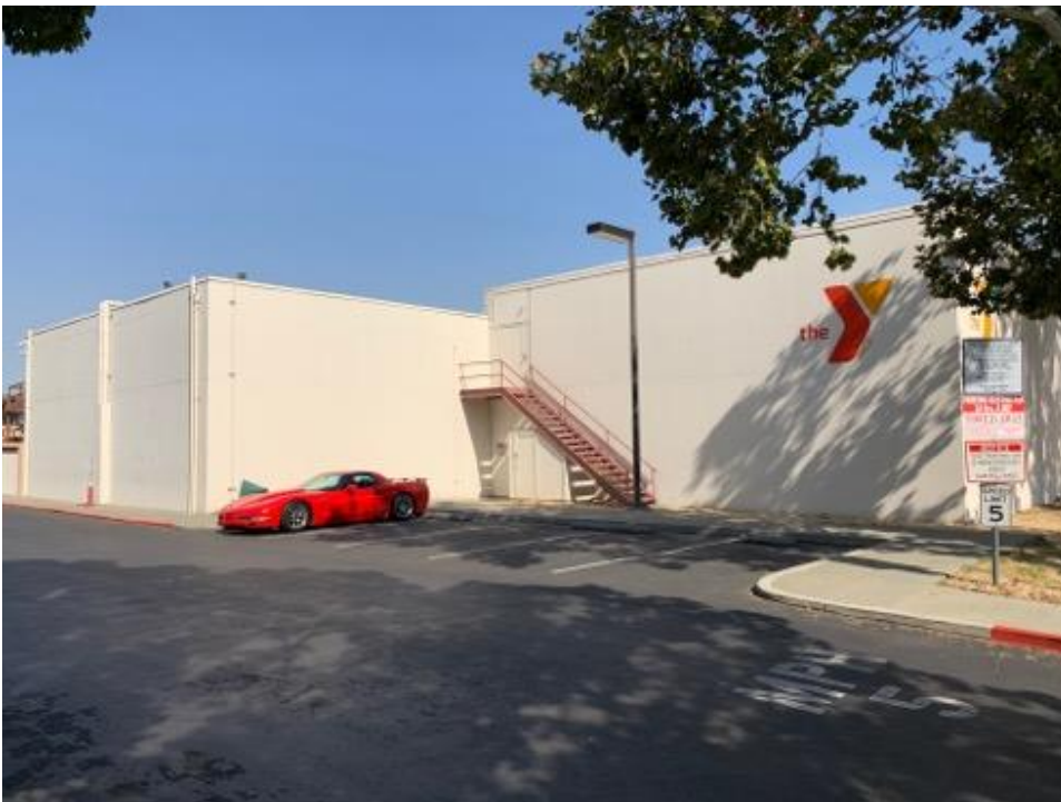
Figure 5. Partial west elevation showing rear of YMCA facility
