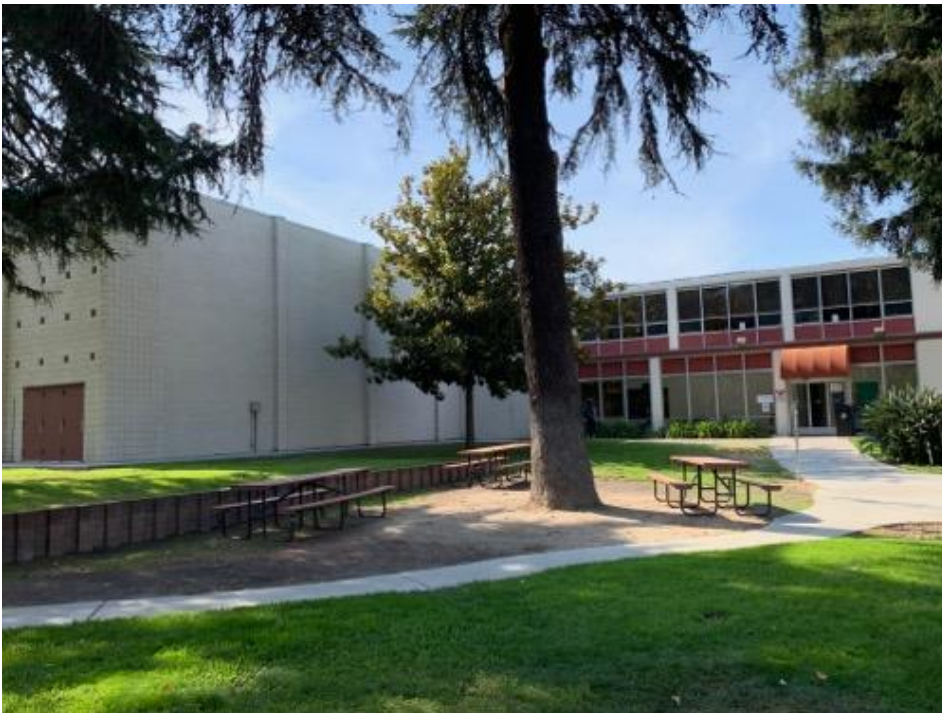
Figure 1. Partial east elevation and main entry
