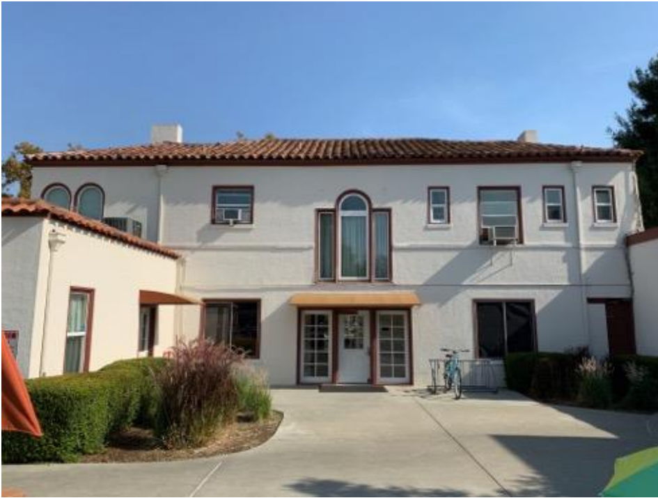
Figure 12. West elevation of administration building
