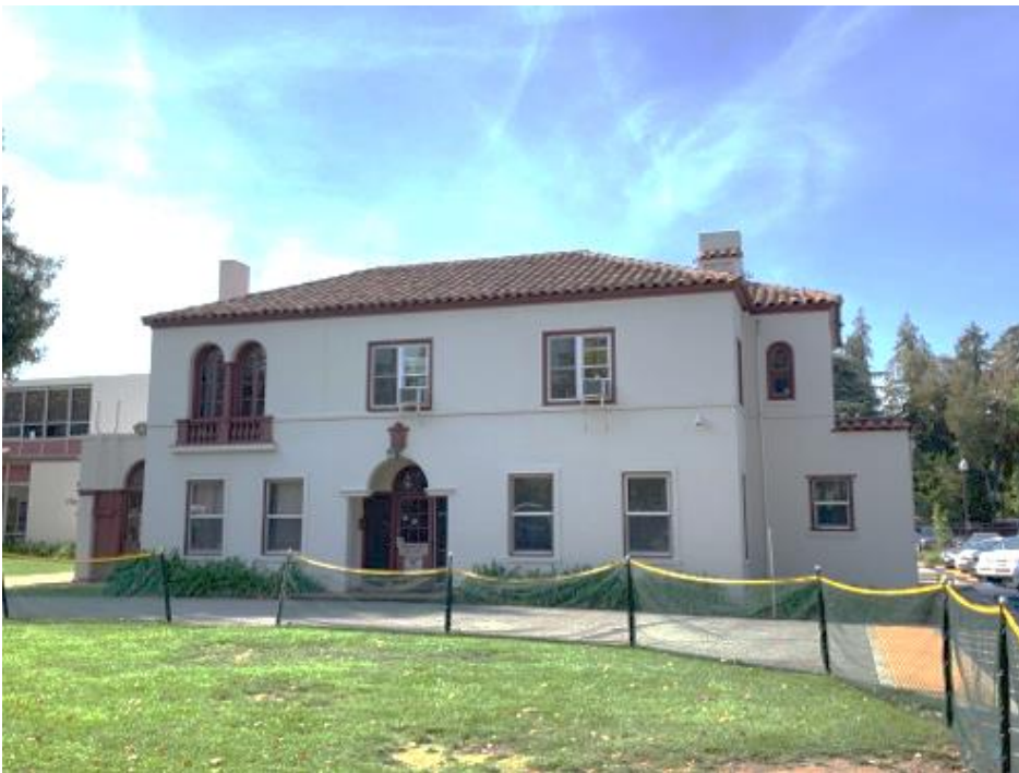
Figure 9. East elevation of administration building
