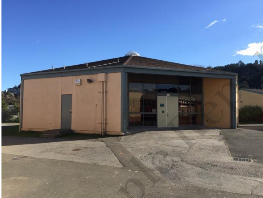
Music Building (1972), looking south
