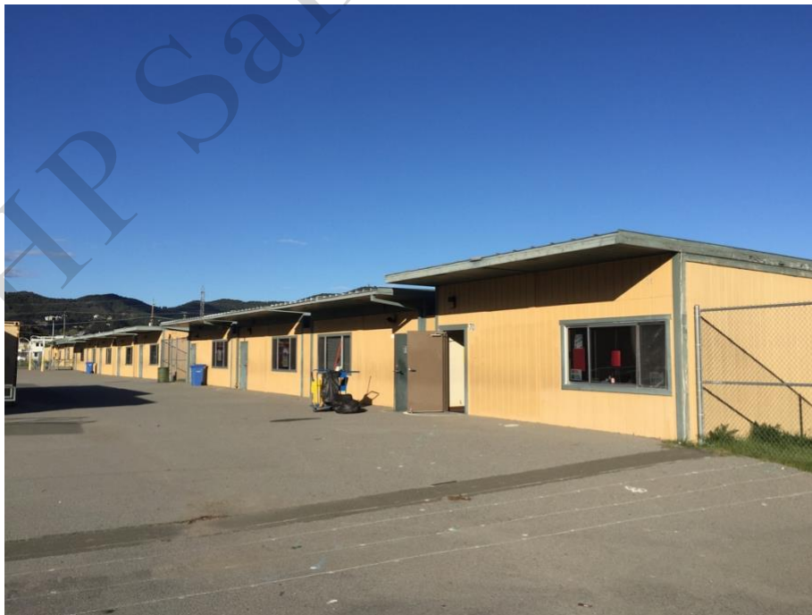
Portable/Relocatable Classrooms (1995), looking northeast
