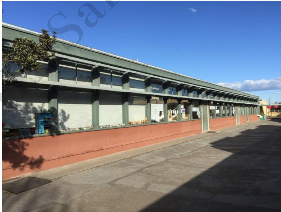
Back of 20s Classroom Wing, looking northeast
