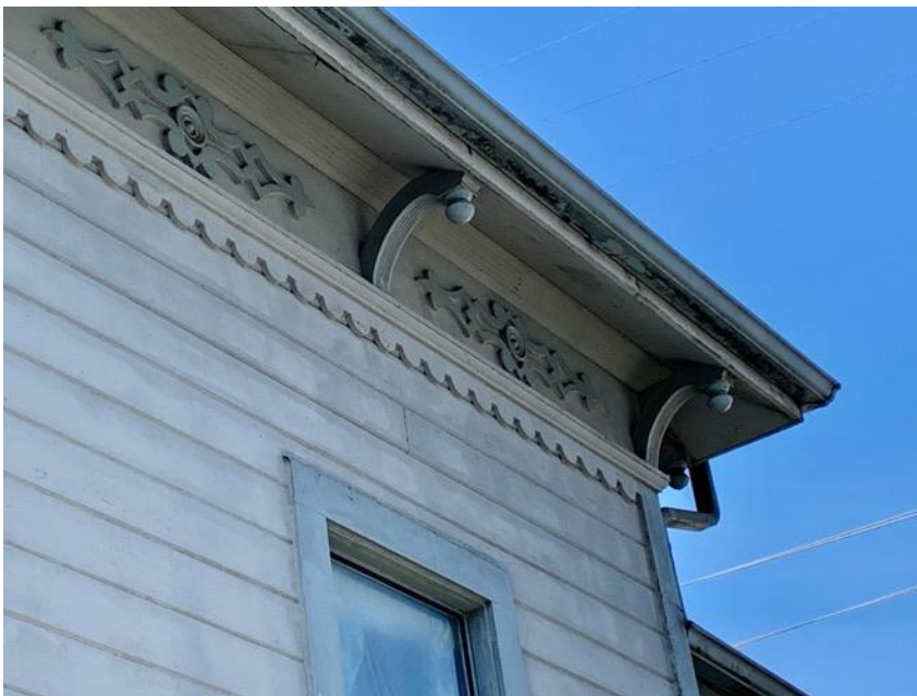
Figure 4. Partial east elevation - cornice detail view
