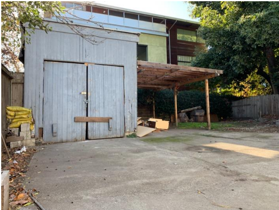
Figure 7. Detached garage and carport at rear of property
