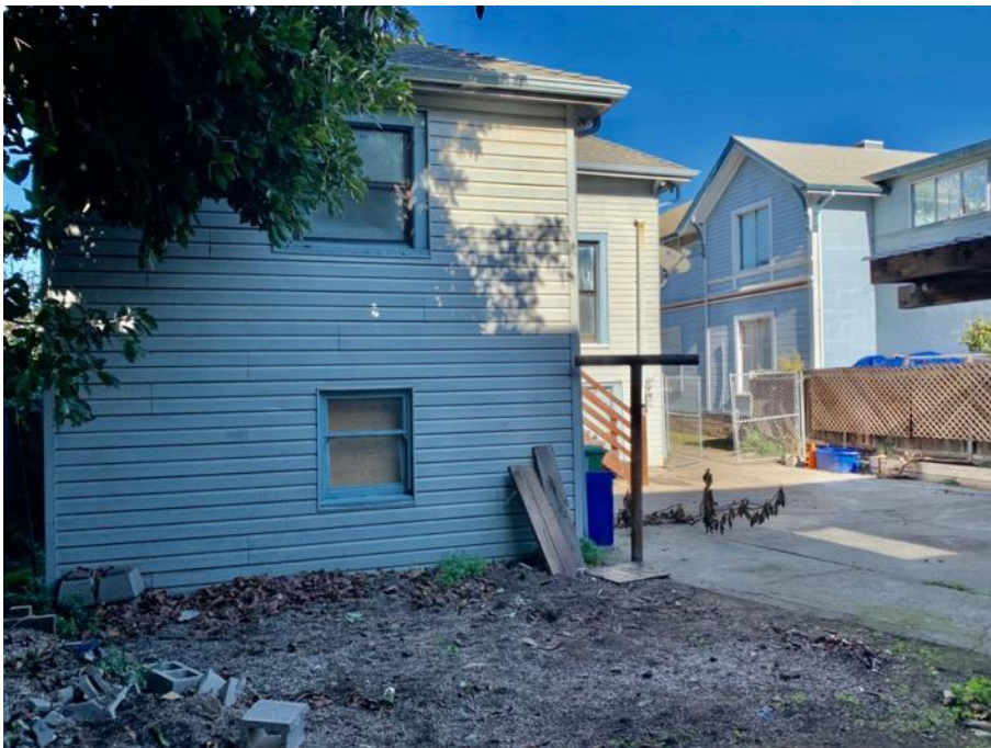
Figure 6. South elevation showing rear addition
