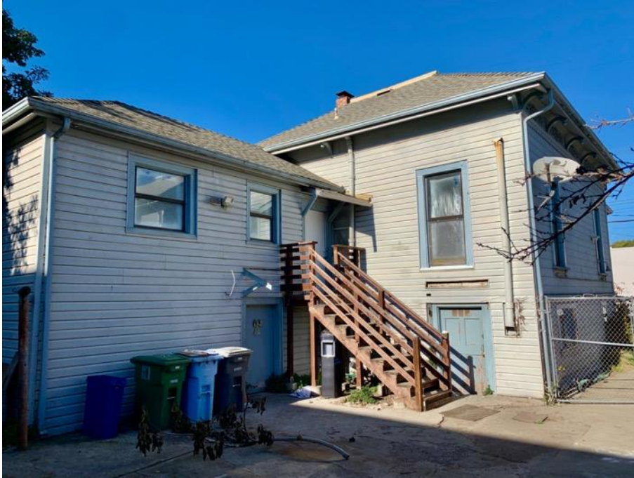
Figure 5. East and partial south elevations showing rear addition.
