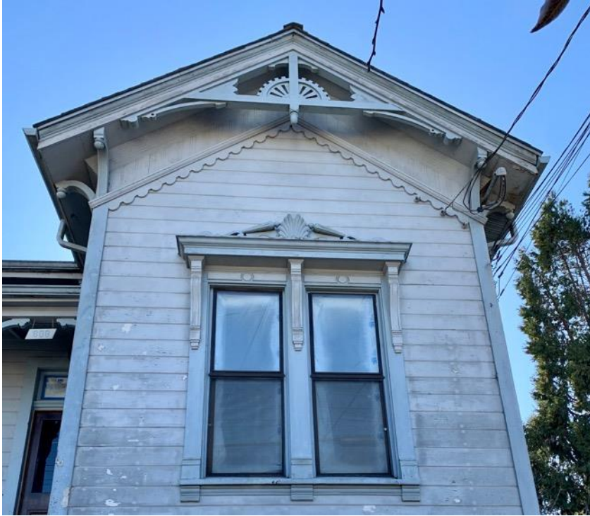
Figure 3. Partial north elevation - ornamental woodwork detail view.
