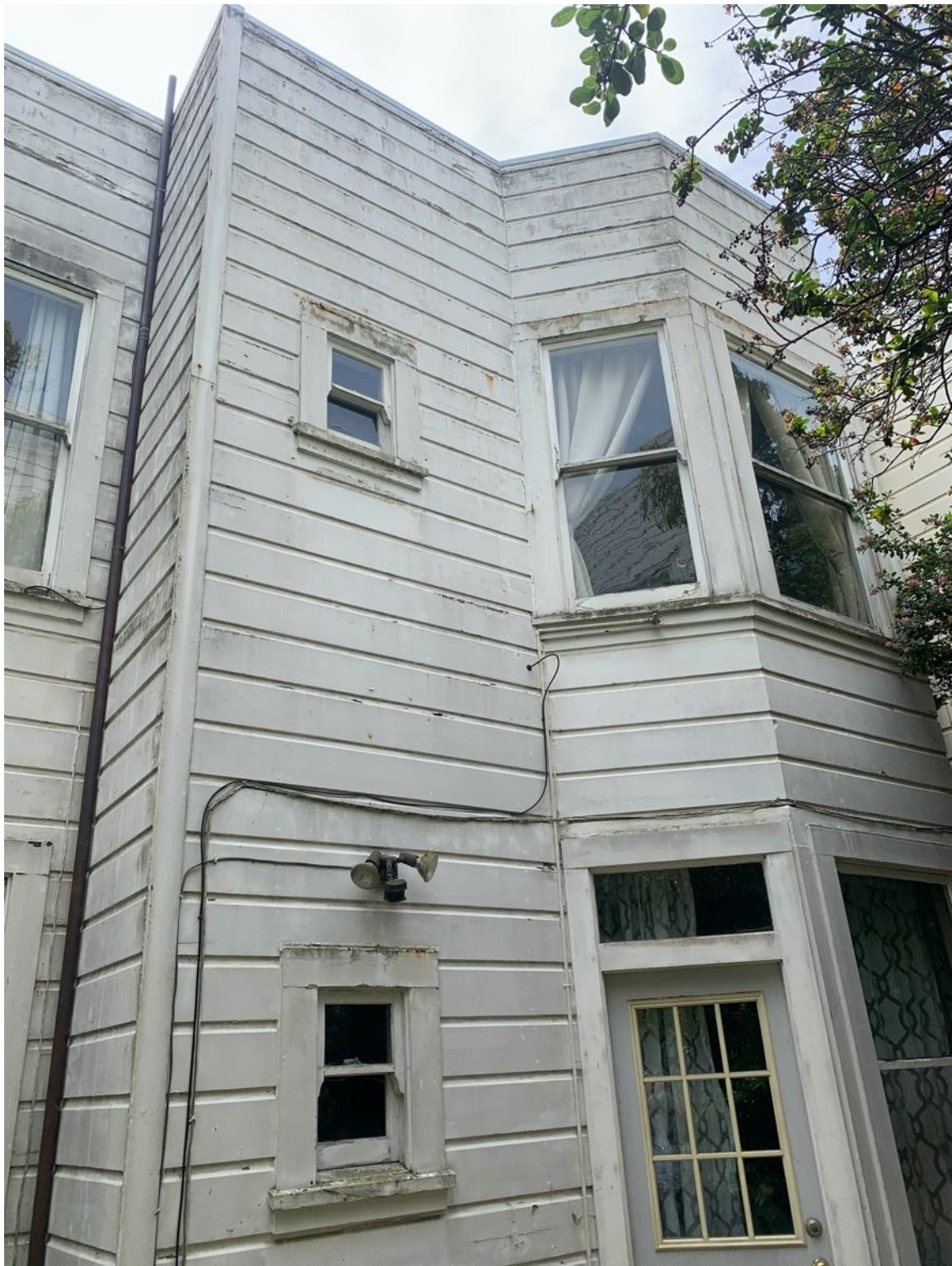
3312-14 Clay Street. Partial View of North-Facing Rear Elevation, Looking Southwest
