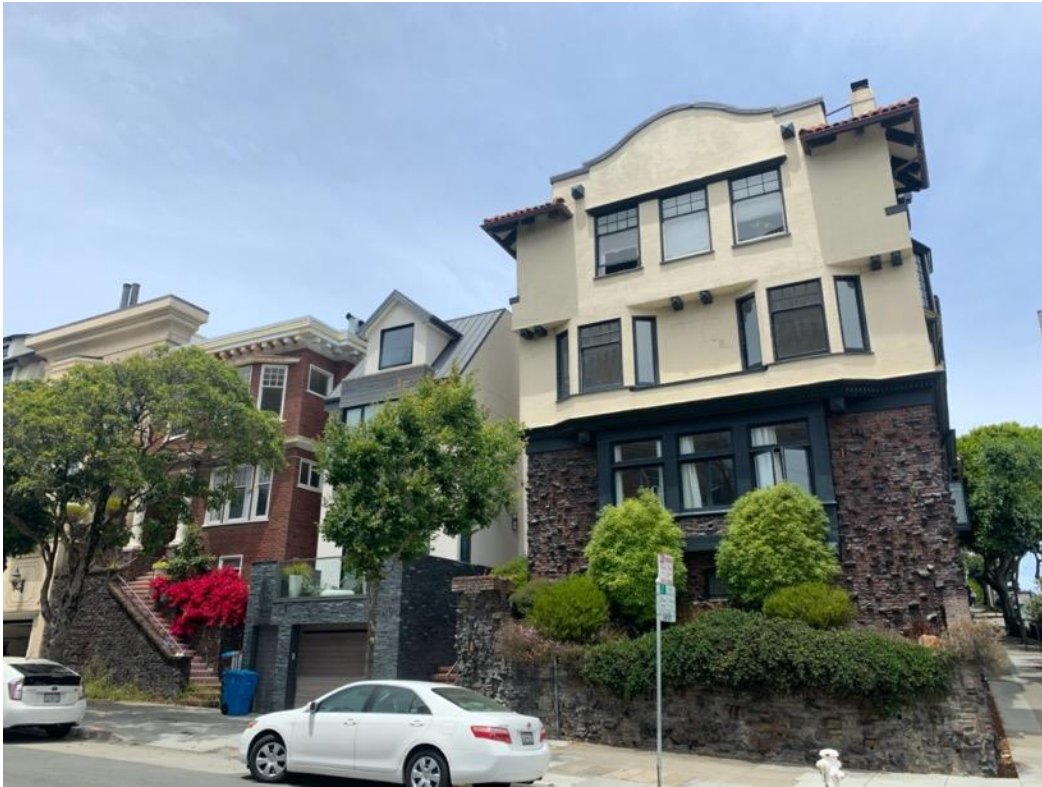
Context View of Clay Street Looking Northwest. 3312-14 Clay Street on left
