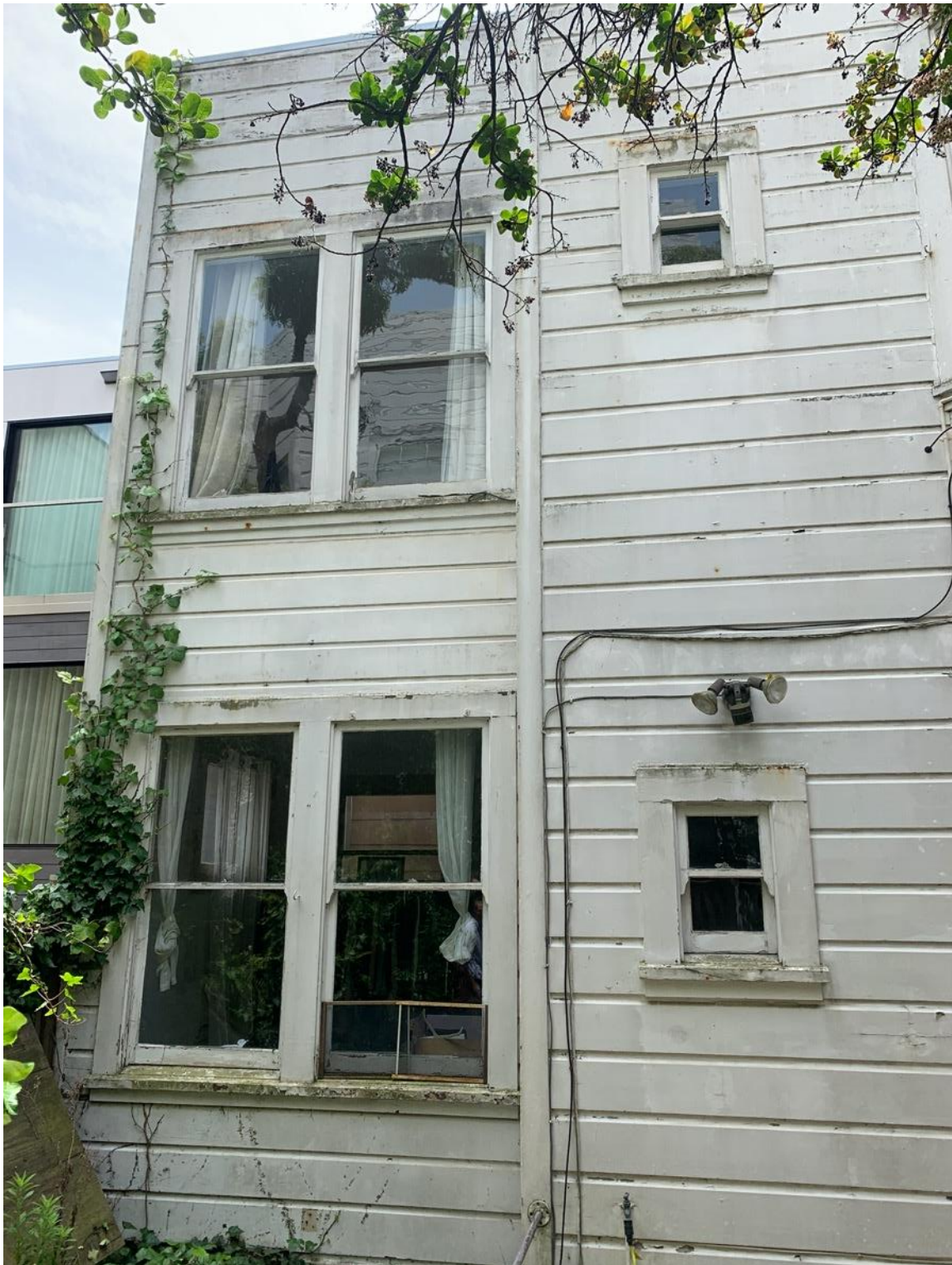
3312-14 Clay Street. Partial View of North-Facing Rear Elevation, Looking South
