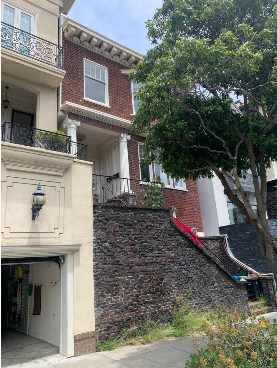
3312-14 Clay Street. View of South-Facing Front Façade, Looking Northeast
