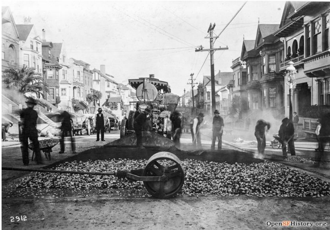
View Looking East on Clay Street at Walnut Street. Street Being Paved. 1915
