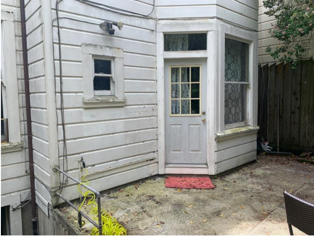
3312-14 Clay Street. Partial View of North-Facing Rear Elevation, Looking Southwest
