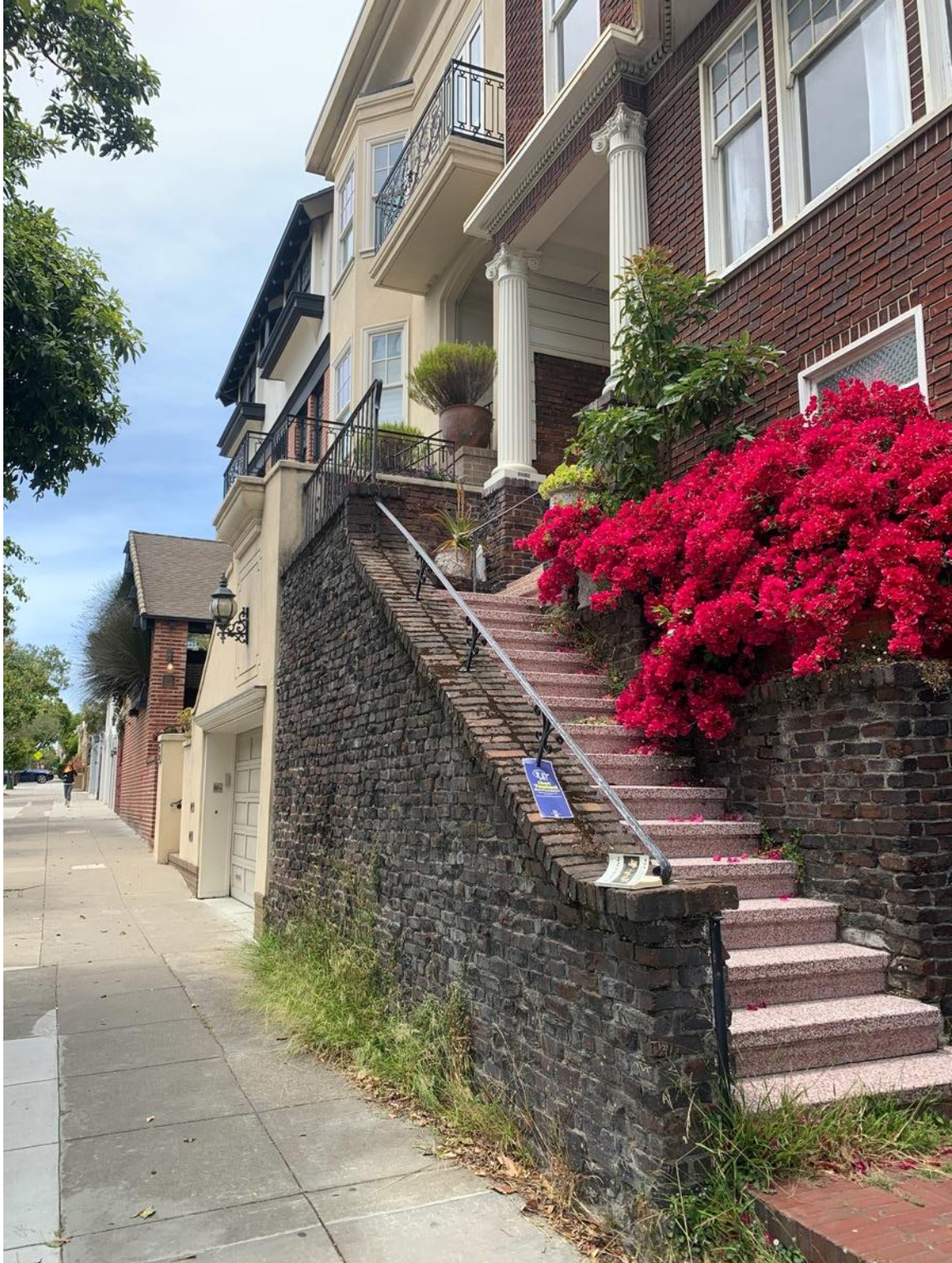
3312-14 Clay Street. Detail View of Clinker Brick Base and Terrazzo Steps. South-Facing Front Façade, Looking Northwest
