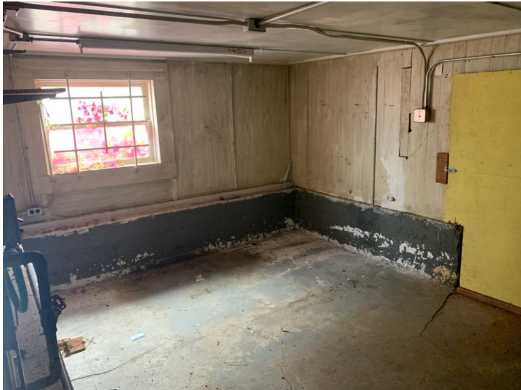
3312-14 Clay Street. Interior View of Basement Level Storage Room, Looking Southwest
