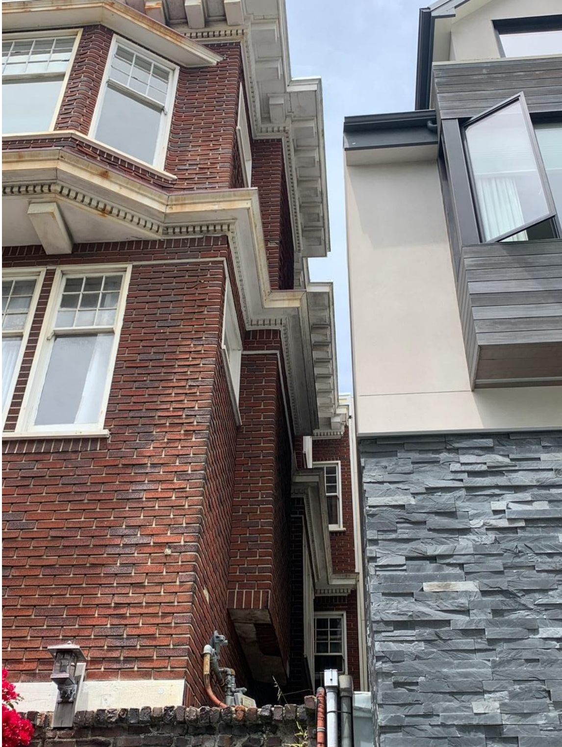
3312-14 Clay Street. Partial South and East-Facing Elevations, Looking North
